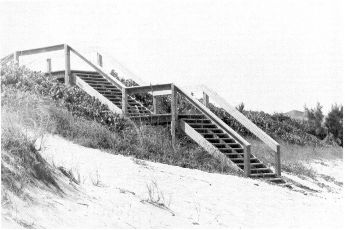
Figure 8.—A dune crossover on Palm Beach sand provides beach access but primarily serves as a form of erosion control to insure dune stabilization.
